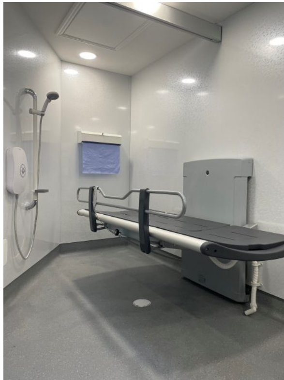
Above: The CP facility includes height-adjustable basin, adult changing table, and ceiling track hoist system.
