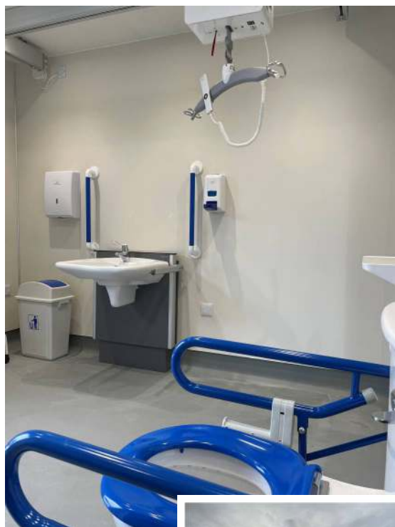
Above: The CP facility includes height-adjustable basin, adult changing table, and ceiling track hoist system.
